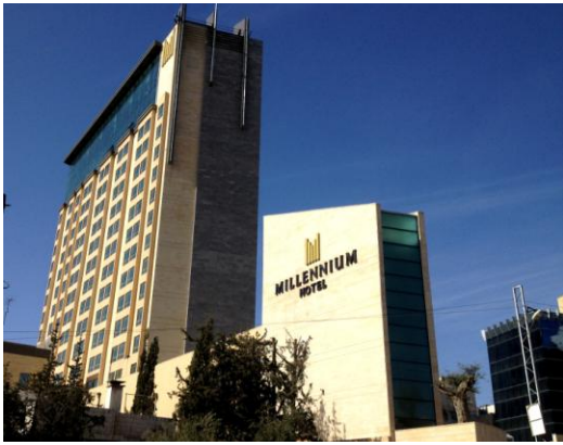
The Millennium Hotel in Amman, for which R&M provided and implemented cabling
