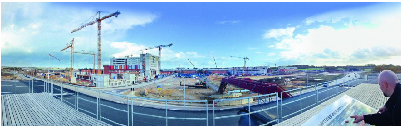
The cabling installation on site
